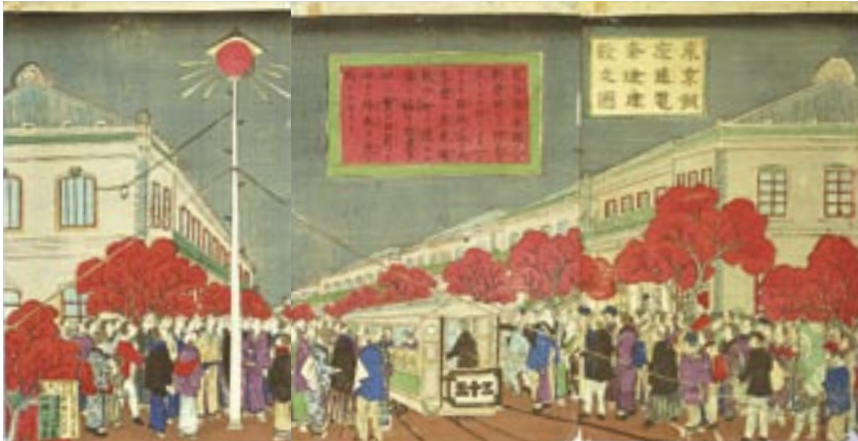
■4J-04 東京銀座通電気燈建設之図 Tokyo Ginza-dori denki-to kensetsu no zu Installing Electric Lights in the Streets of Ginza, Tokyo
