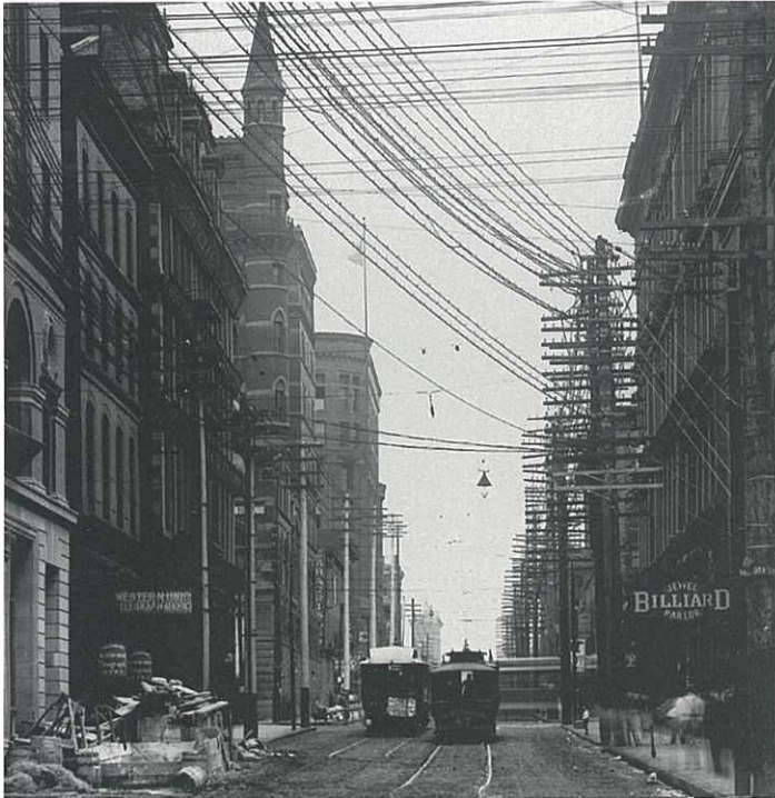
Early telegraph, telephone and electrical lines in a typical American city, ca. 1910.
