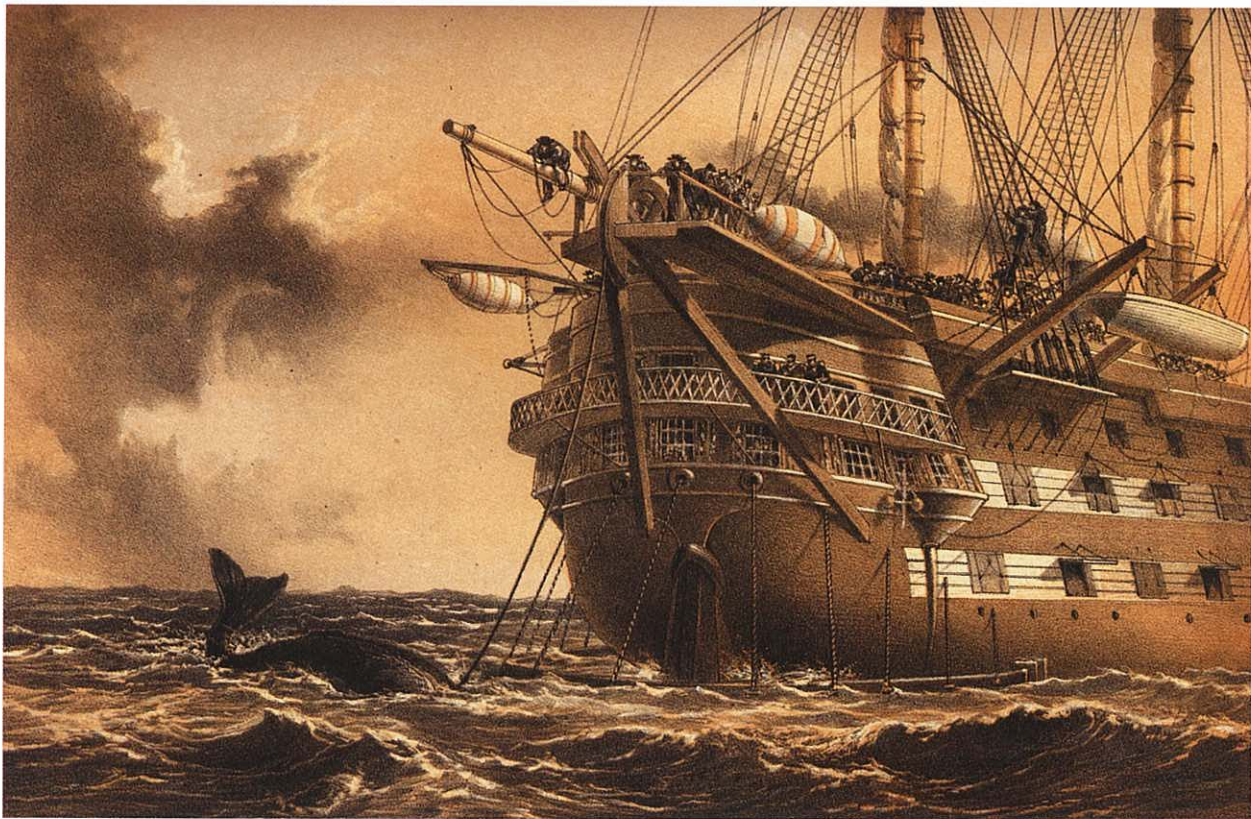
"Laying the Atlantic Cable," lithograph, 1866
